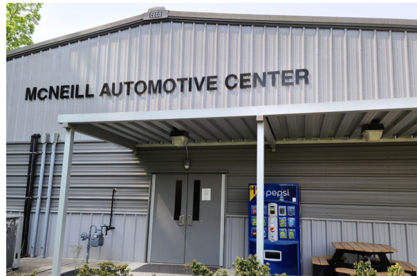
Automotive Complex: 2013 Collision Repair: Shop and Paint 4,260 SF McNeill Automotive: Shop, Offices 10,920 SF
