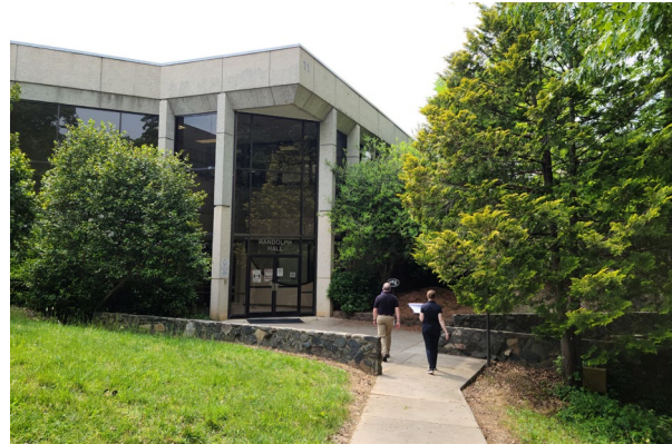
Randolph Hall: 1978 Wilkes Early College High School, Gymnasium 31,310 SF
