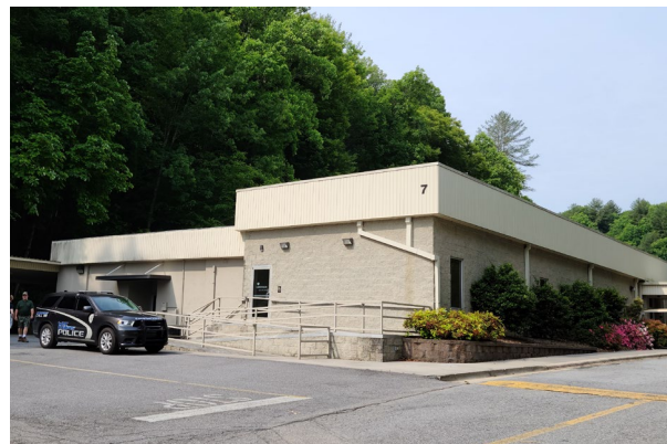
Building 7: 1978/2010 Campus Police, Offices, Shipping and Storage 7,619 SF
